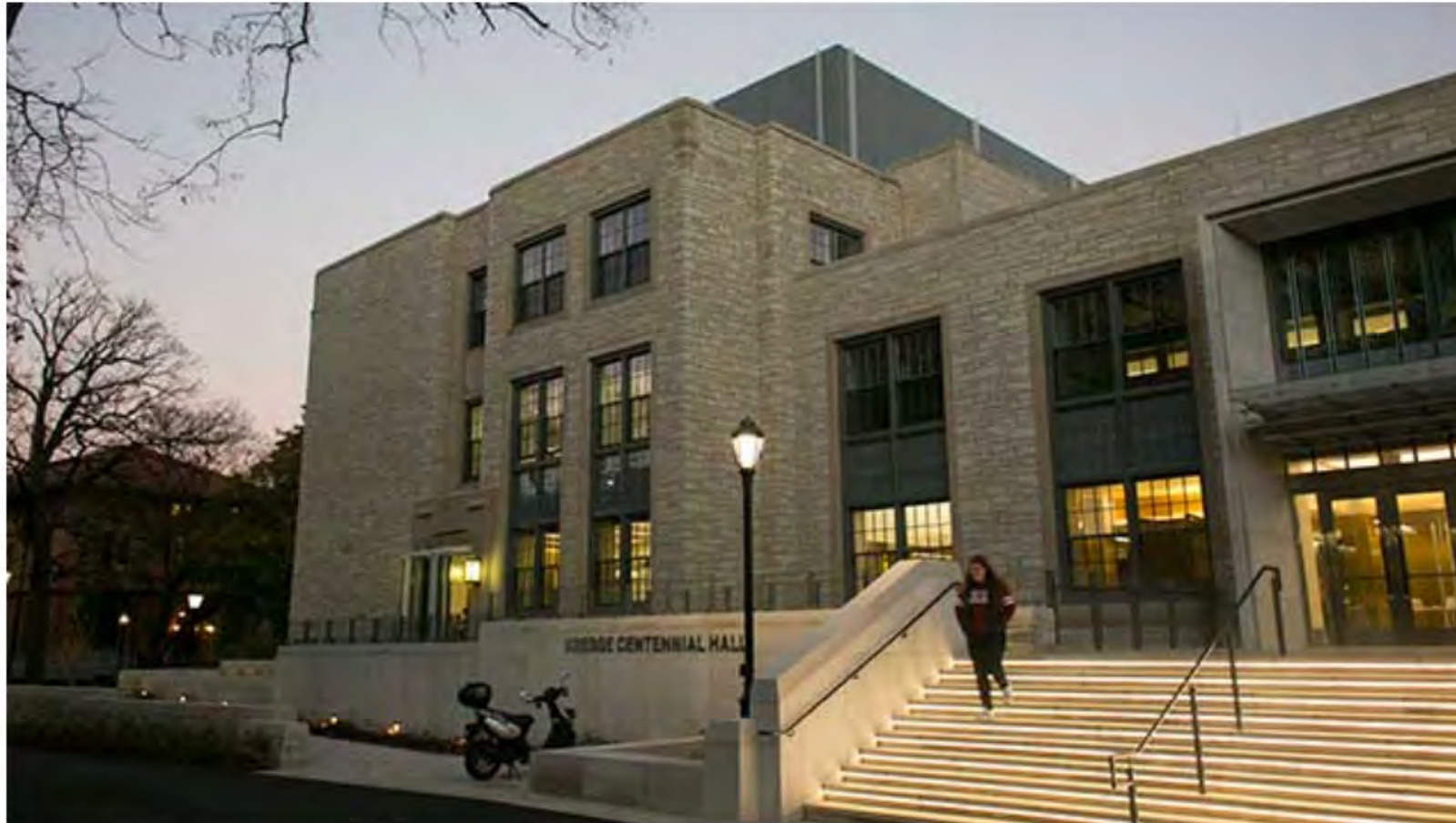
Kresge Hall is the first University building to be certified as LEED Platinum. The 63-year-old academic building reopened in August 2016 following two
